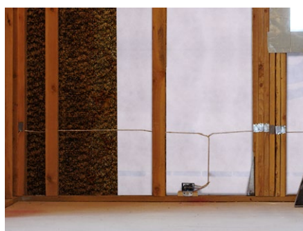
Drainage Mat with Watergate Plus installed.
