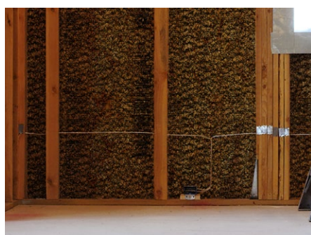
Drainage Mat installed, ready for underlay.
