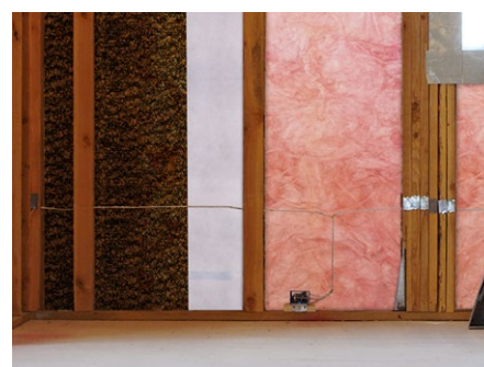
Drainage Mat with wall lining and insulation.
