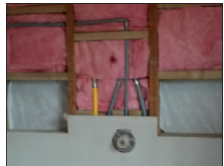
Completed with wall lining and insulation
