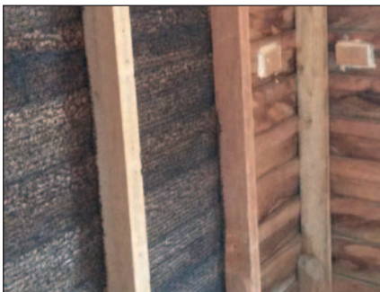
Drainage Matt WaterWay 9714M installed ready for underlay
