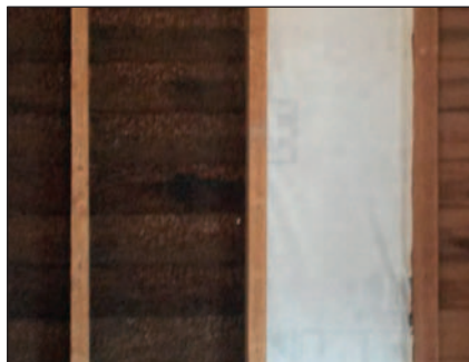
Drainage Matt WaterWay 9714M with Watergate Plus installed
